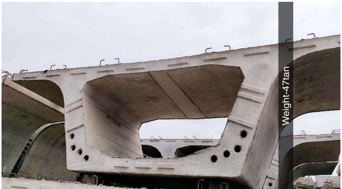
Figure 4: weight of 1 casted segment
