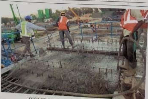
SEGMENT CONCRETING OF DECK SLAB
