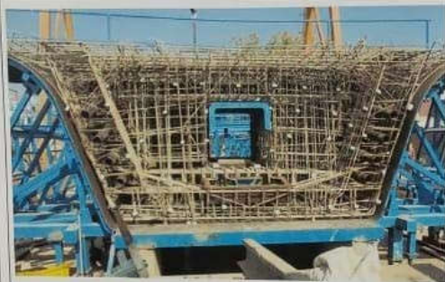
SEGMENT CABLE PROFILING
