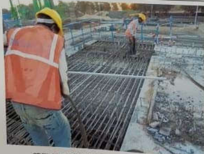
SEGMENT CONCRETING OF DECK SLAB
