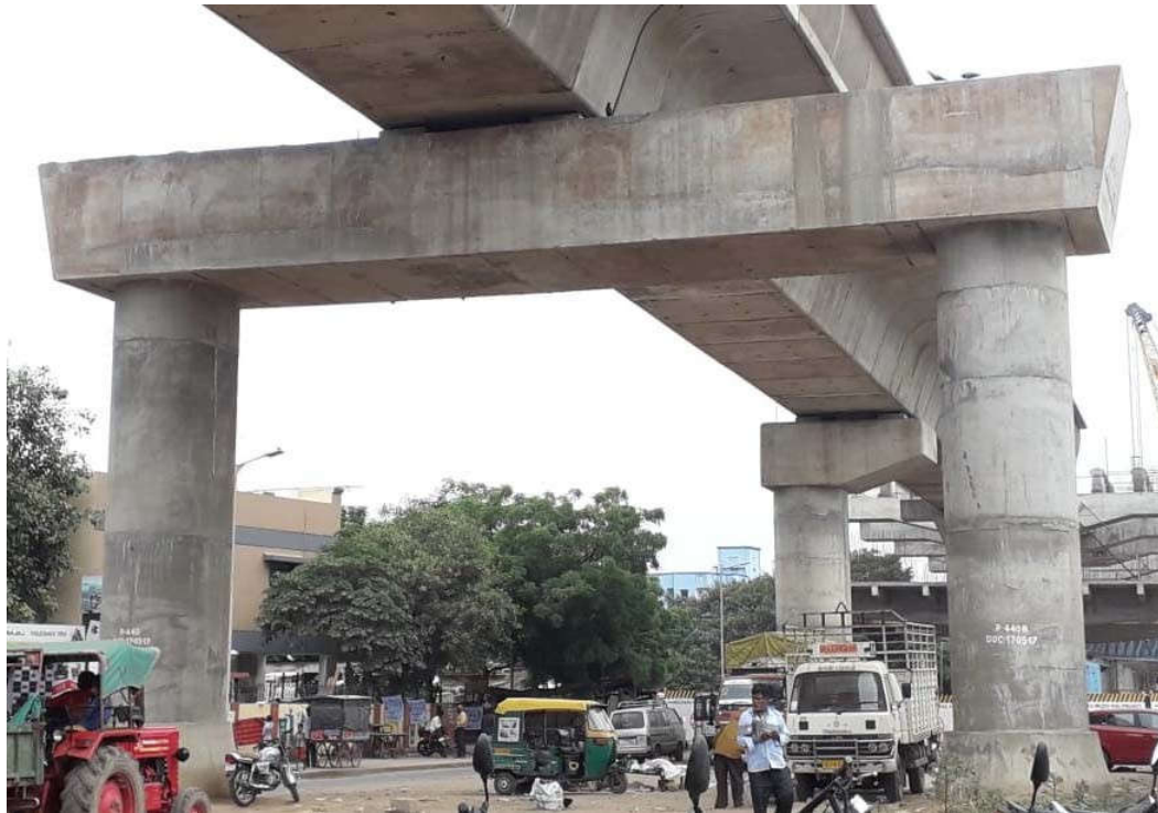
Figure 6: Portal beam and crash barriers
