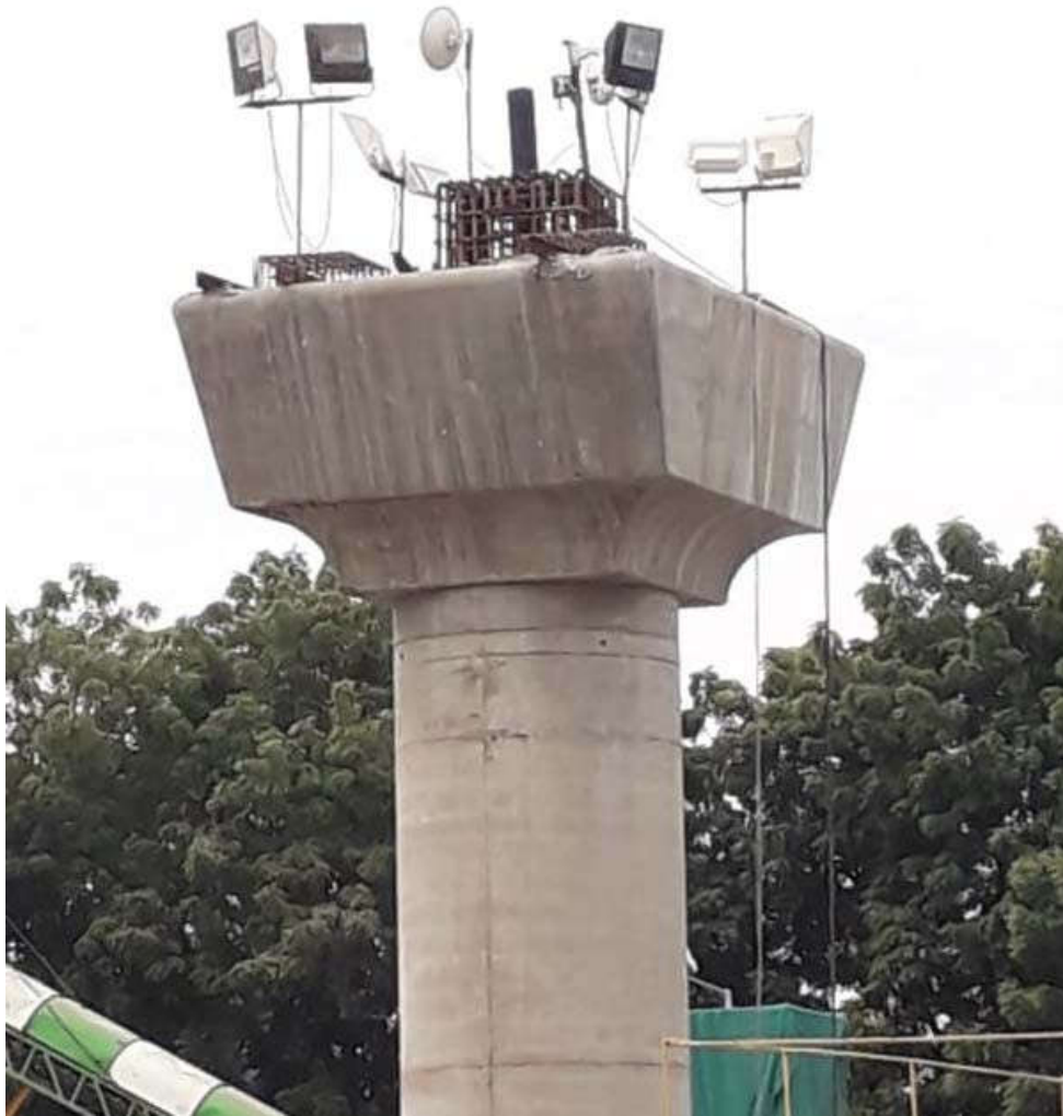
Figure 5: Shear key and pedestal
