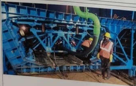
SEGMENT CONCRETING OF SOFFIT
