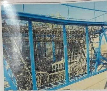
SEGMENT RIENFORCEMENT WORK IN ZIG
