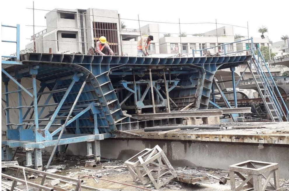
Figure 1: Casting of segments
