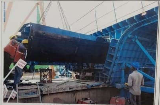
SEGMENT INNER TROLLEY FIXING
