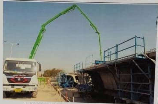
SEGMENT CONCRETING BY BOOM PLACER
